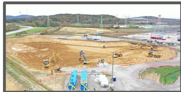
PORTS Site Deactivation and Demolition Program Activities
