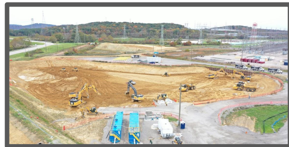
PORTS Site Deactivation and Demolition Program Activities
