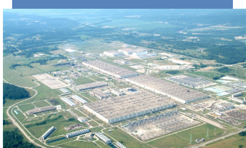
Historical aerial view of the PORTS site. Photo credit: U.S. Department of Energy
