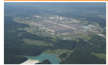
Photo: US Department of Energy (DOE)
