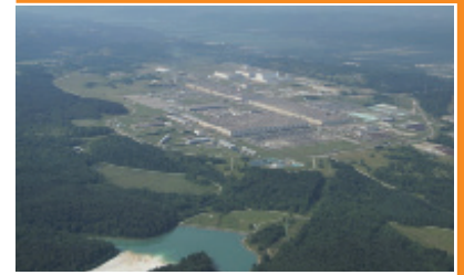
Photo: US Department of Energy (DOE)
