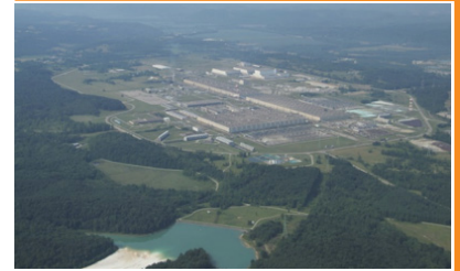
Photo: US Department of Energy (DOE)
