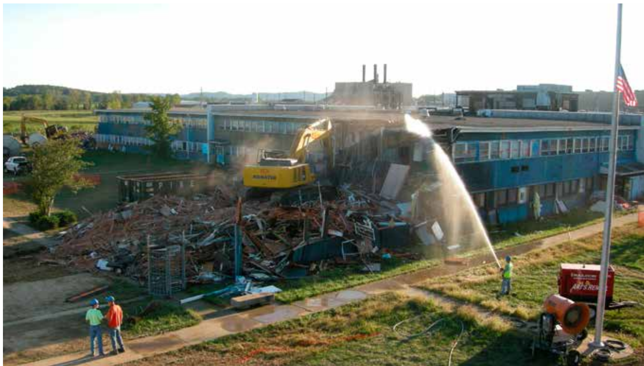
Demolition of the X-100 Building
